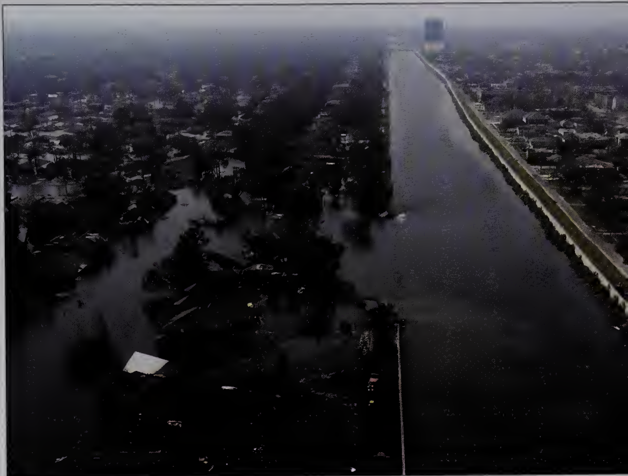
A canal breached, New Orleans
